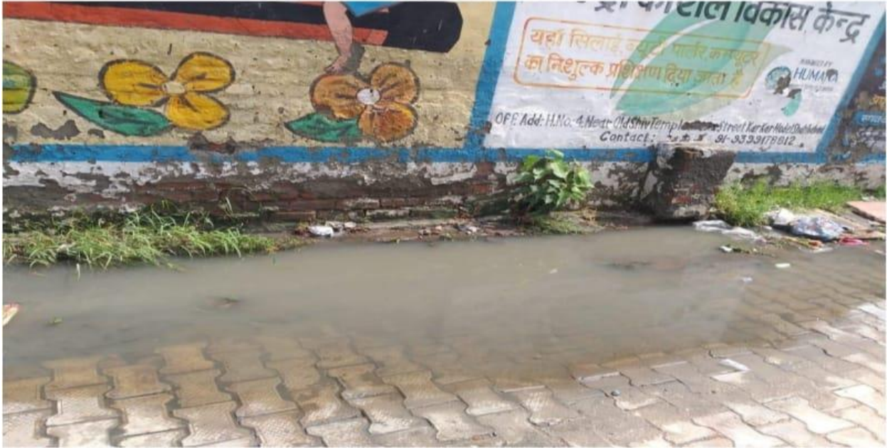
Overflowing drains in Karkarmodel
